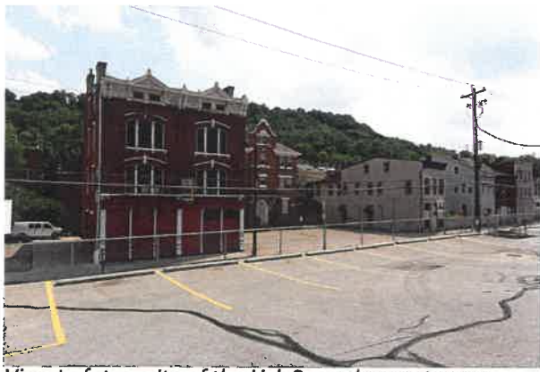
View to future site of the Lick Run urban waterway
