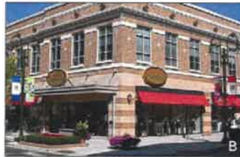
Low density mixed-use building
