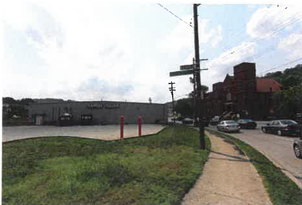
Backside of Family Dollar, northern edge of Lick Run urban waterway
