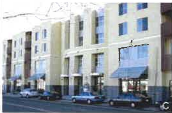
Medium density mixed-use building
