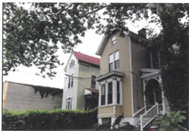
Housing on Carll Street in North Fairmount
